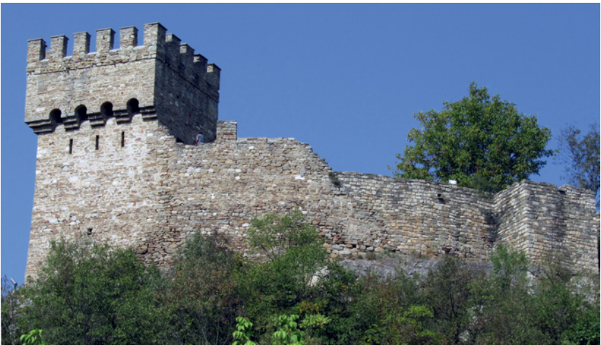
FIGURE 12 "The tower of Baldwin", seen from outside. AUTHOR'S PHOTO.
